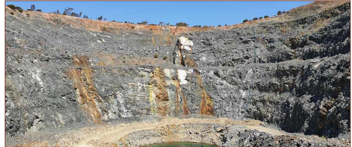
Residual nickel sulphide mineralisation in the southern wall of the 132N Open Pit.
