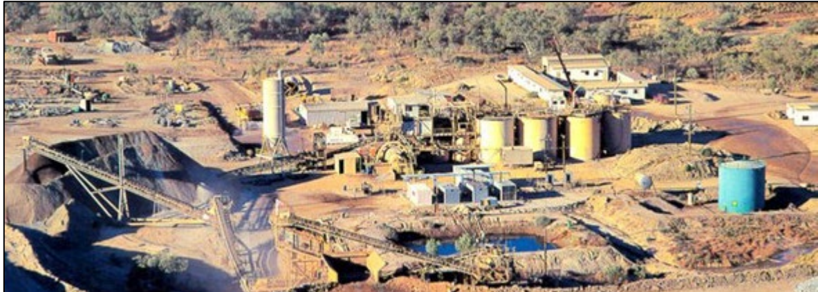
Figure 7: Butchers Creek gold processing plant. Circa 1996.
