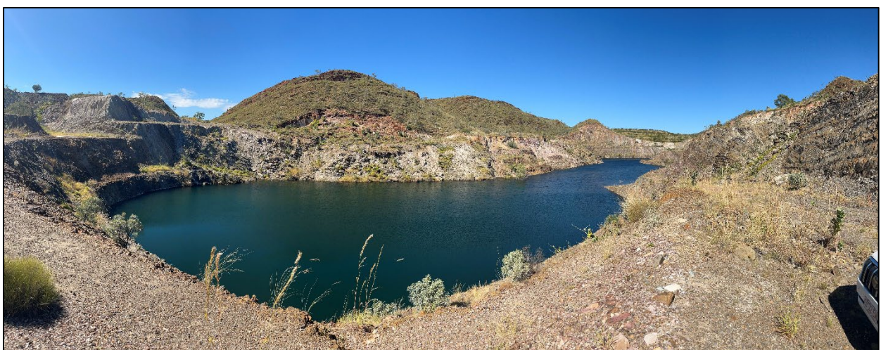
Figure 3 - Butchers Creek open pit May 2024
