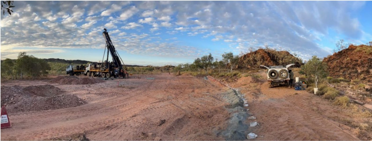
Figure 5: Drilling underway at Butchers Creek
